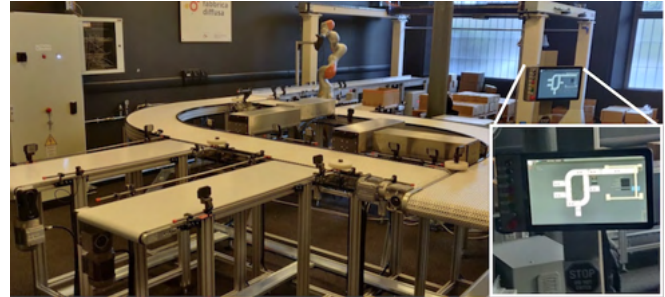
(a) The conveyor belt system transports packages loaded by a gantry (top center) to two bays (bottom left); a graphical Human-Machine Interface (right) is currently used to control the system.
